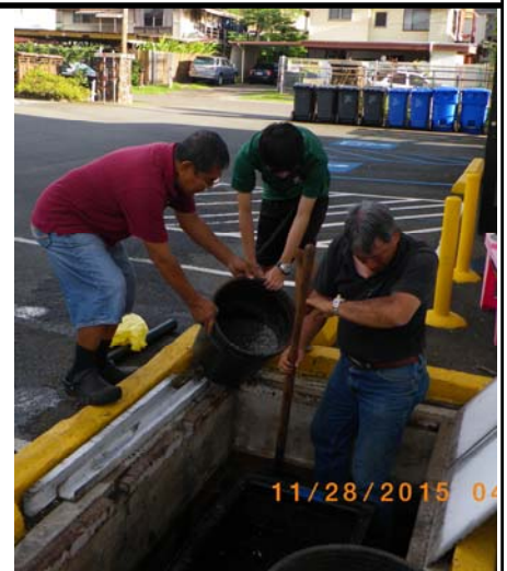
Working on the Preschool Grease Pit! Thank you for doing the "dirty" work ♥
